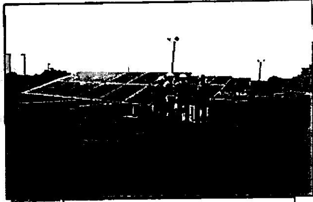
Solar PV Plant in Ash Pond.
